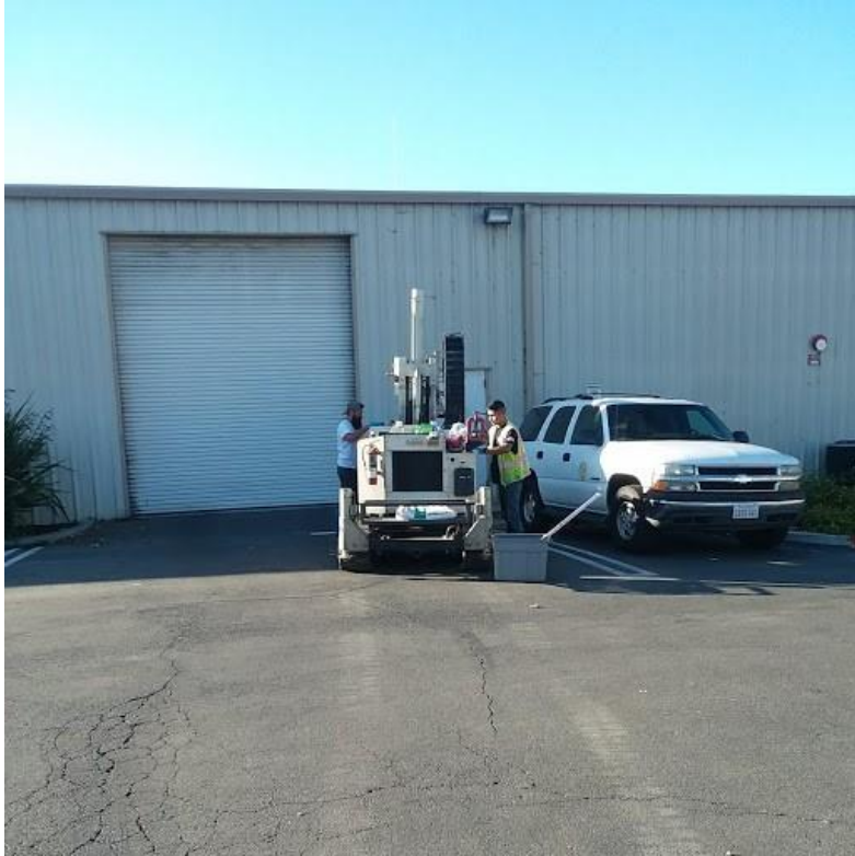
Photograph 1: View of the soil boring activities.
