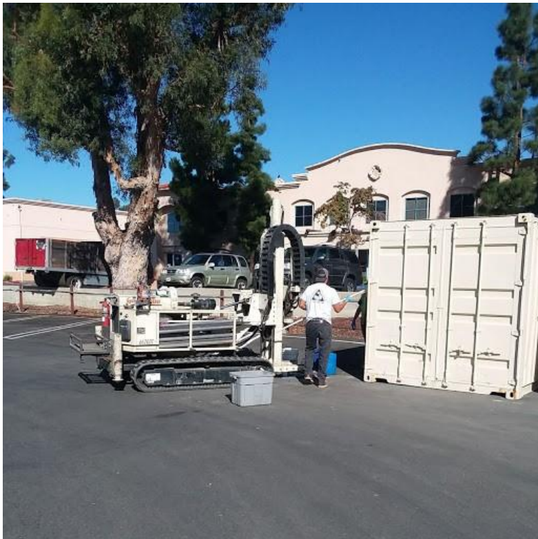
Photograph 2: View of the soil boring activities.
