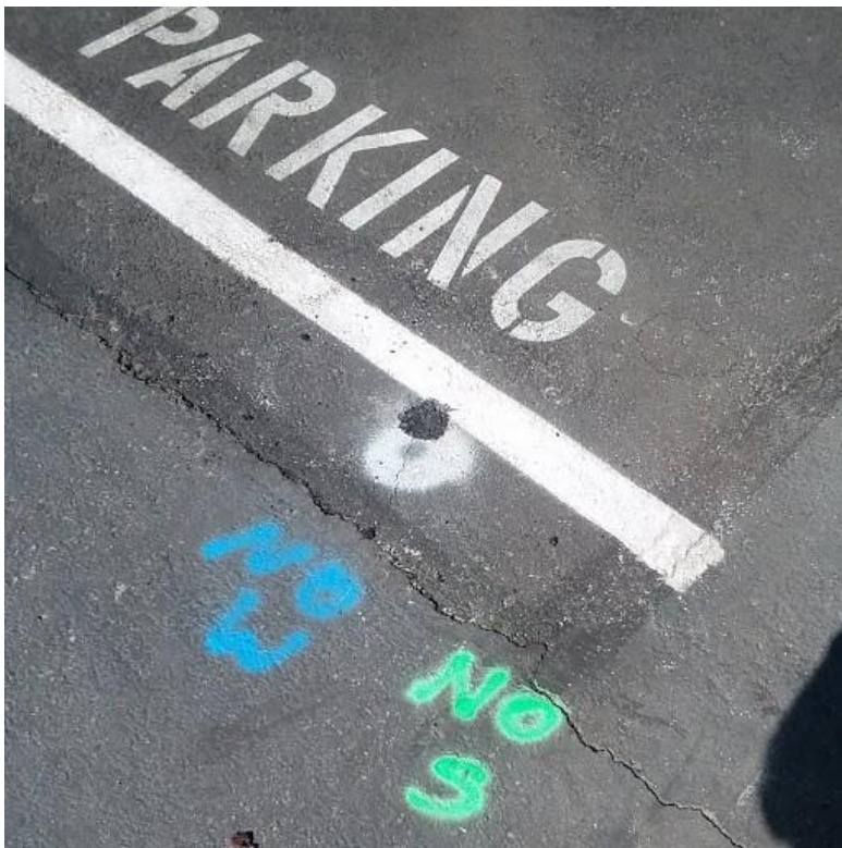
Photograph 4: View of a completed and patched soil boring location.
