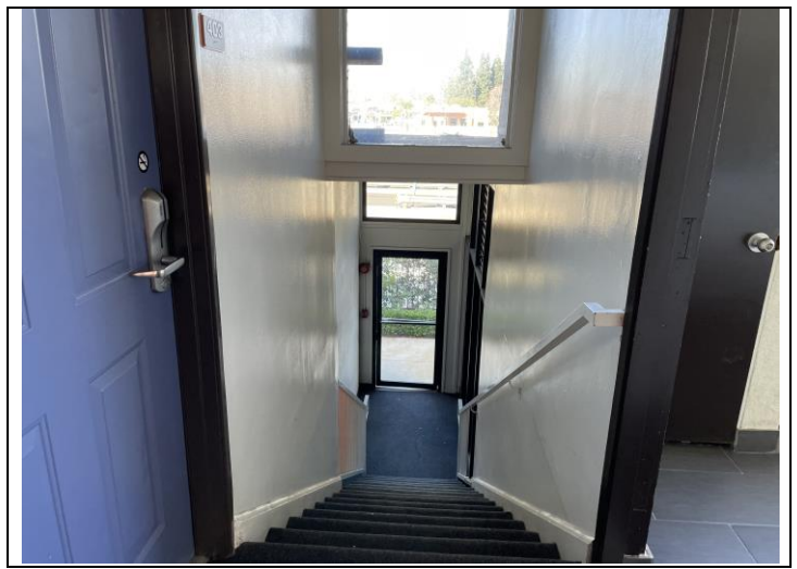
8. View of Building 400 Stairwell.
