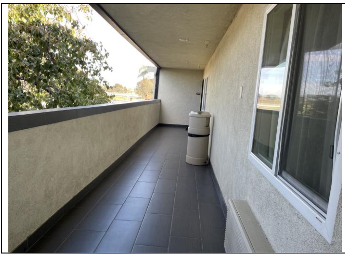
7. View of Exterior Building 400
