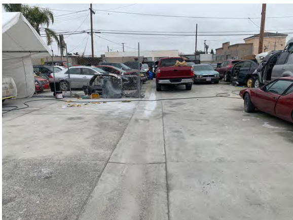
Concrete swale between auto service buildings at 15072 and 15082 Adams Street,
