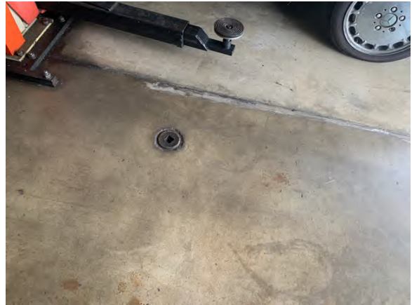
Old floor drain and lift cutout.
