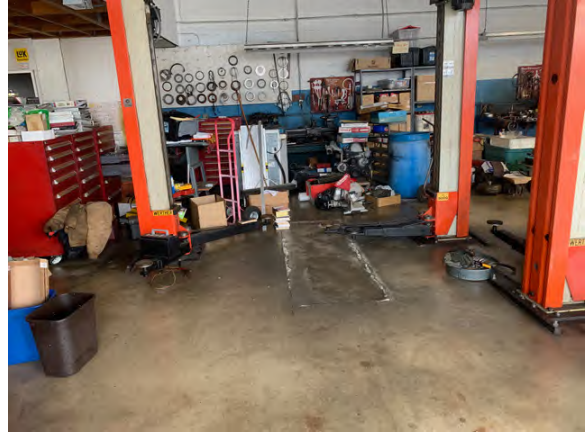
Interior of Reliable Transmissions. Concrete patch evidence of former in-ground lifts.
