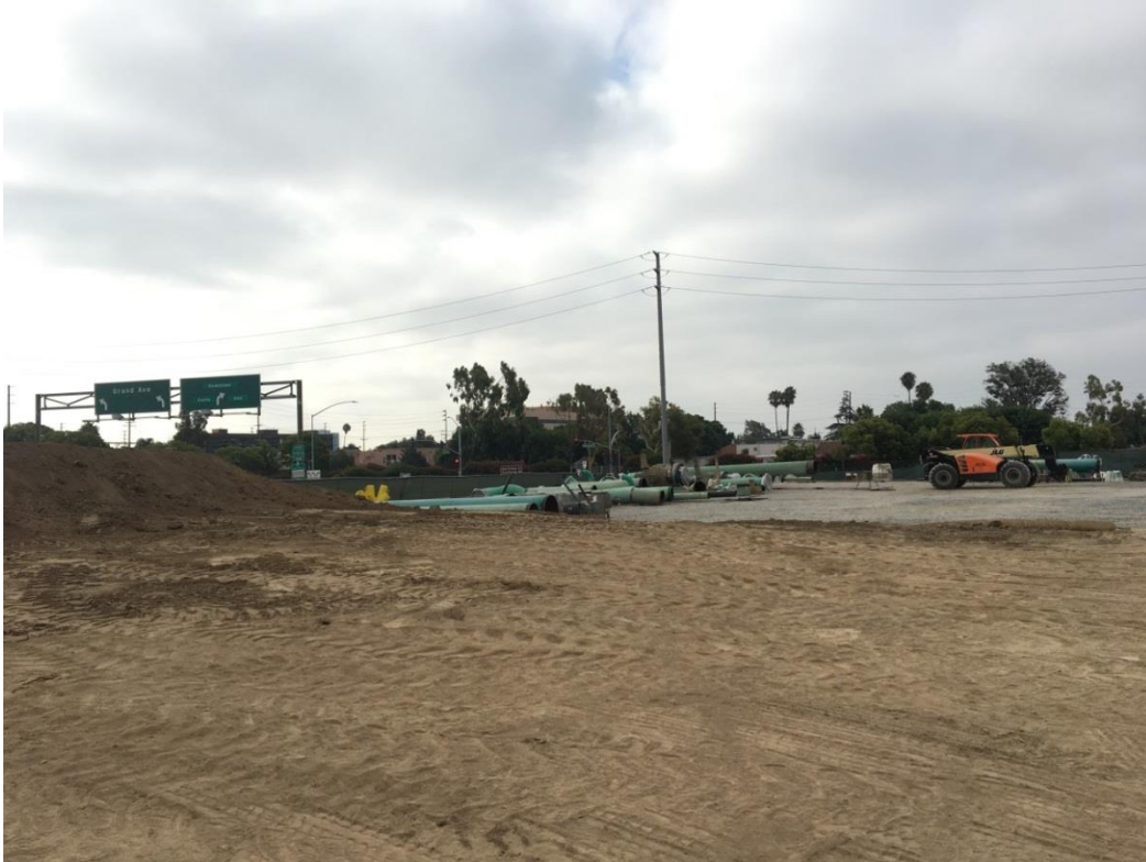
Figure 4 View of Northern Portion of APE (APN 398-092-14), Facing Southeast
