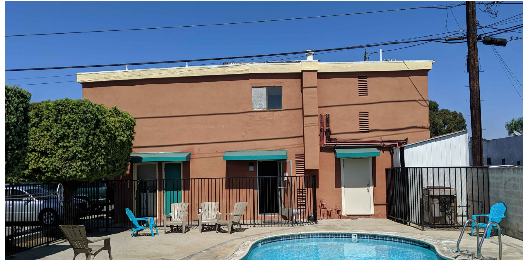
VIEW LOOKING NORTH FROM SOUTHEAST CORNER OF SITE 09
