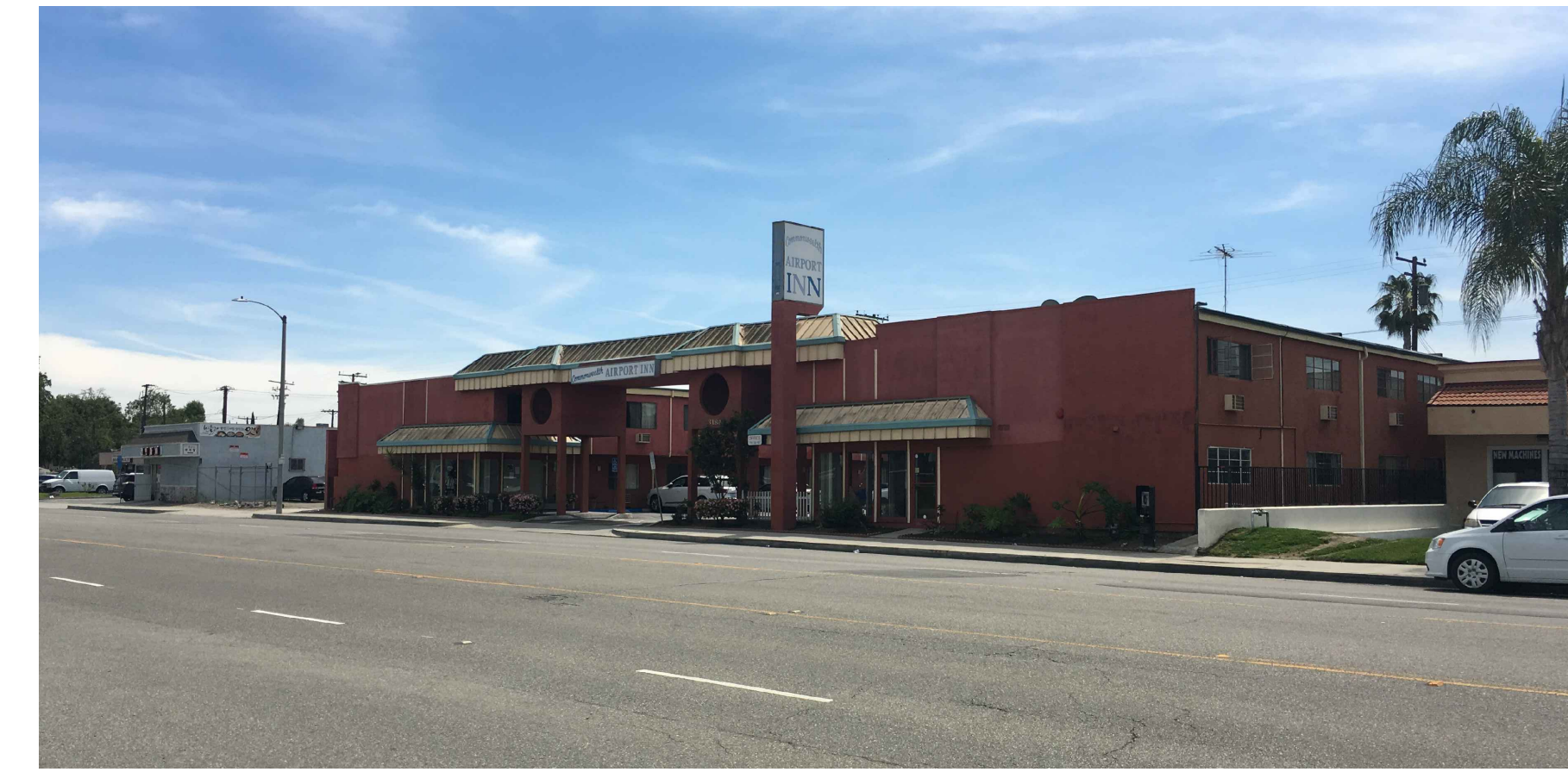
VIEW LOOKING SOUTHEAST FROM COMMONWEALTH AVE. 04
