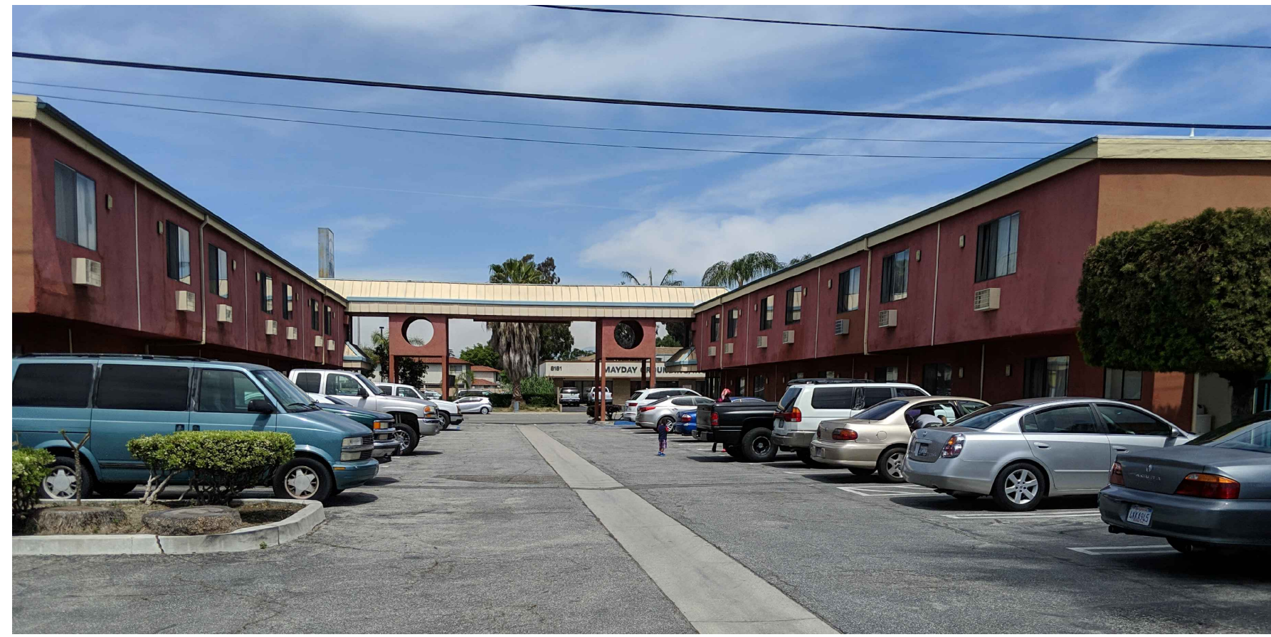
VIEW LOOKING NORTH FROM SOUTHWEST CORNER OF SITE 10
