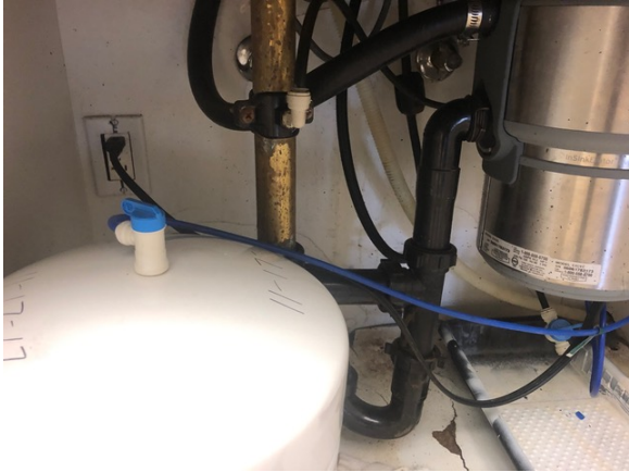
Typical under sink condition, no moisture noted
