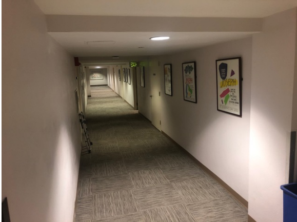
Basement corridor, all substrates are dry
