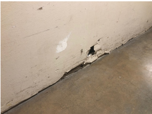
Close-up, dry and not suspected to be water damage related
