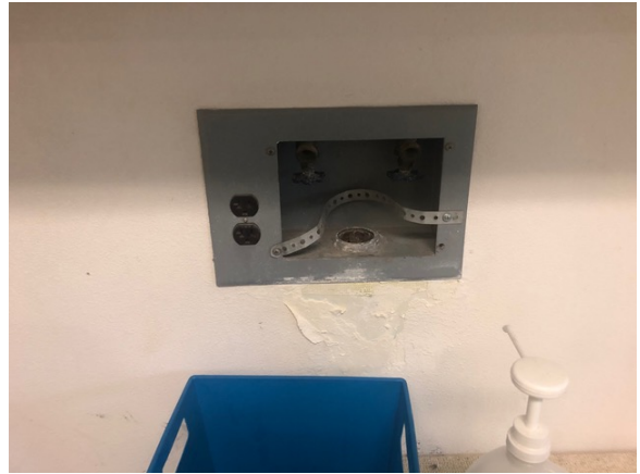
Laundry water connections, no moisture detected
