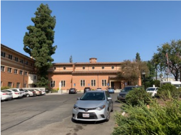
Northern view of the Site from the parking area.
