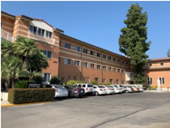
Northern portion of the building at the Site looking northwest.
