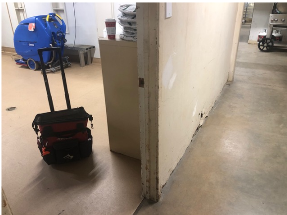
Basement laundry area, damaged portion of the wall at the base was all dry and no surface mold was noted.
