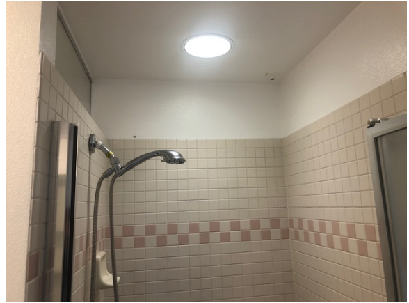
Typical bathroom, no moisture conditions noted
