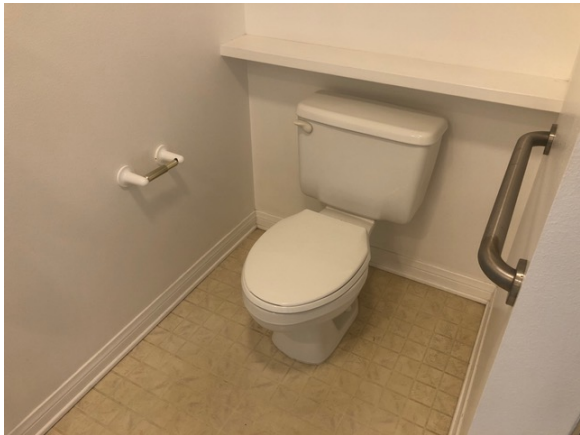
Typical bathroom, no moisture conditions noted
