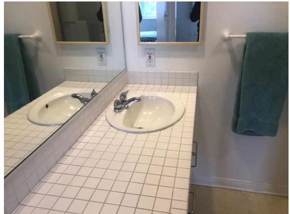
Typical bathroom, no moisture conditions noted
