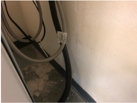
Laundry water connections, no moisture detected
