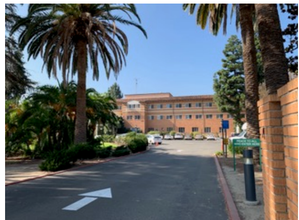
North driveway to the Site from Batavia Street looking west.
