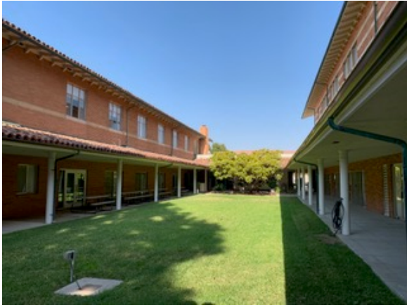
Yard and adjacent University of San Francisco/Sisters of St. Joseph facilities.
