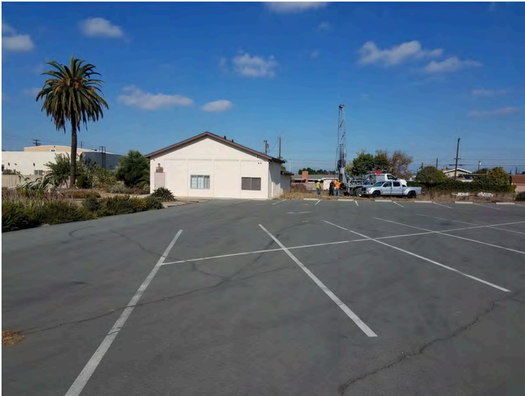
View of third building located along northern Property boundary.
