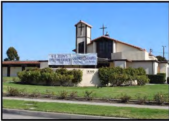
Photo 1: View of church on project site from the Valley View St. eastern frontage road.
