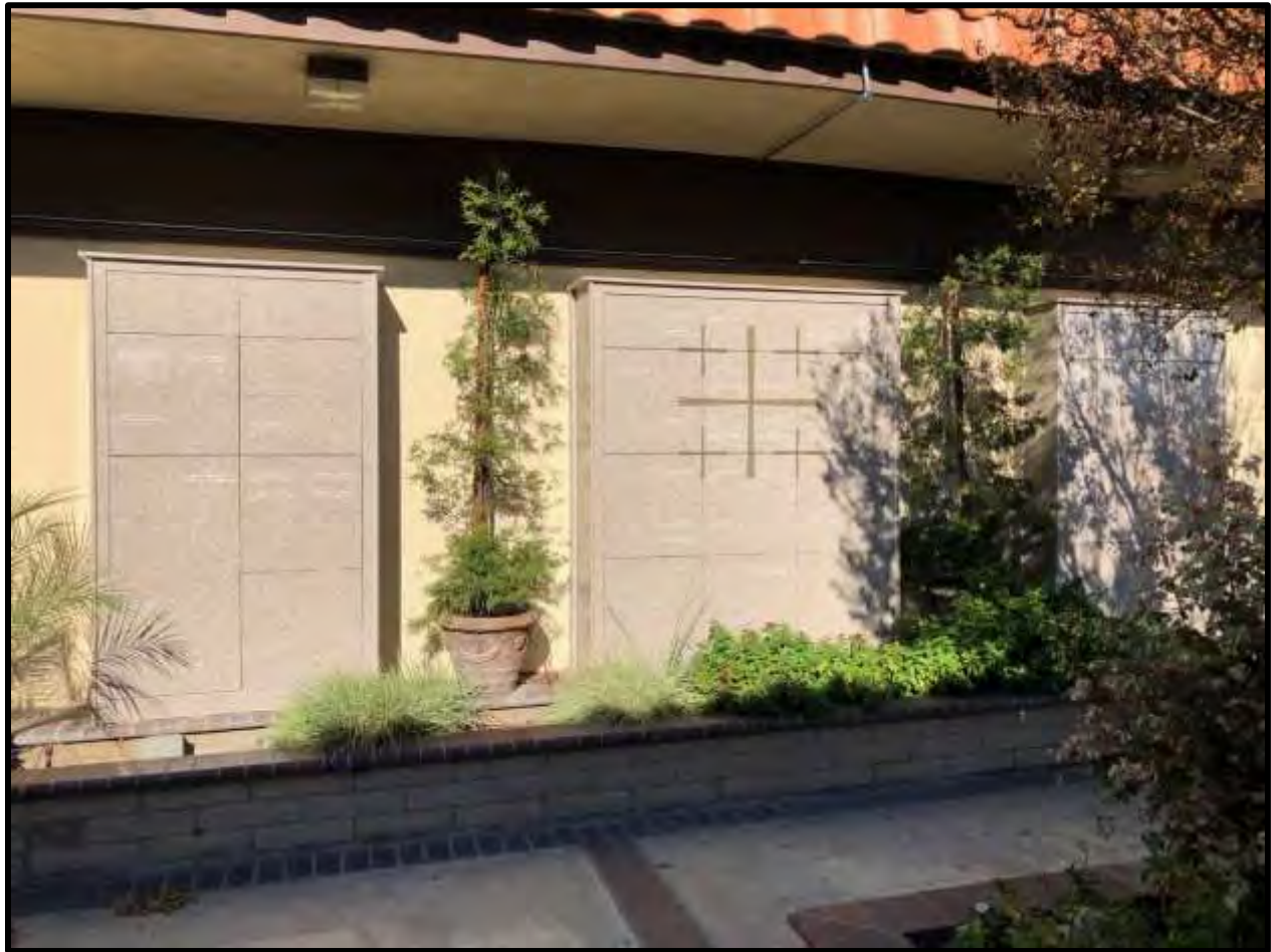
Figure 4.3-7 COLUMBARIUM WALL ON PARISH HALL AND GARDEN; VIEW TO NORTH
