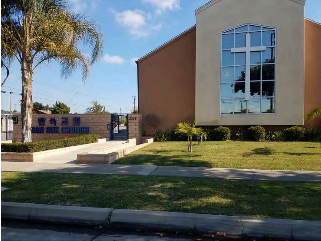
View of northern adjoining church (8246 Valley View Street).
