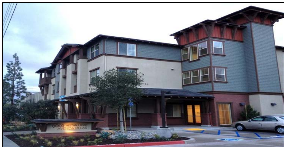
AVENIDA VILLAS AFTER
