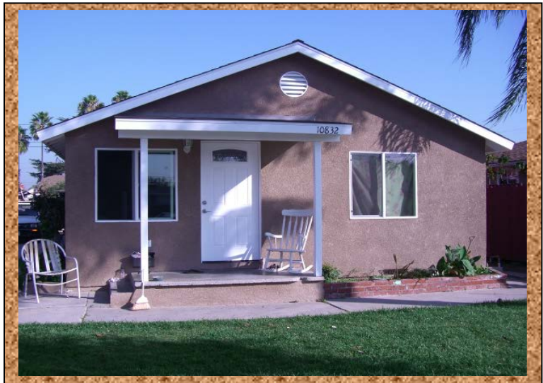
AFTER HOUSING REHABILITATION (ROOF, STUCCO, PAINT) AND LANDSCAPING
