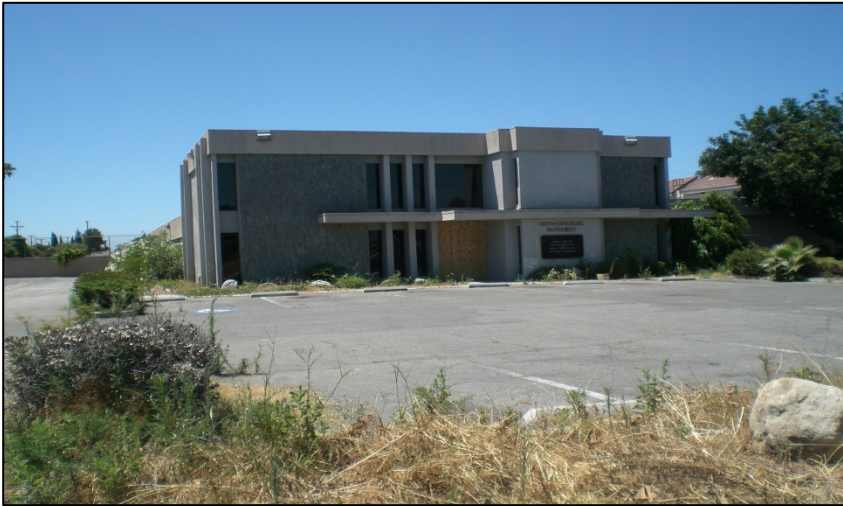
ABANDONED STRUCTURE BEFORE
