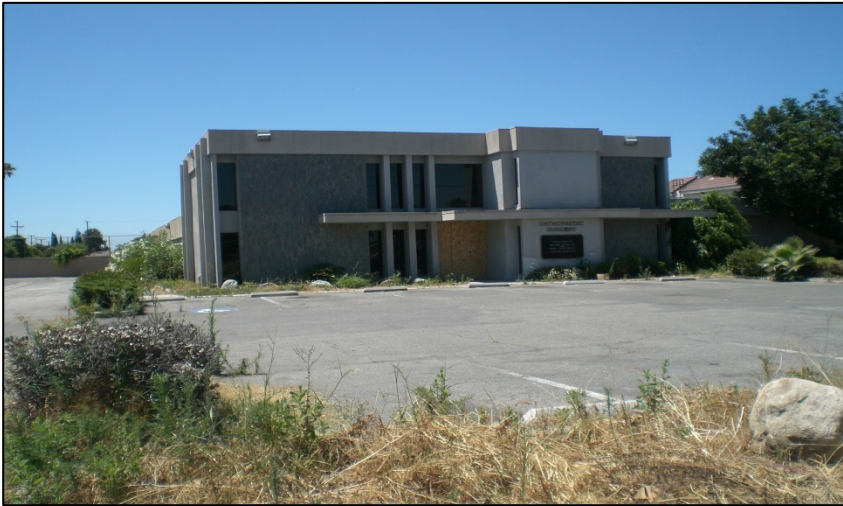
ABANDONED STRUCTURE BEFORE
